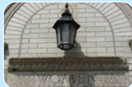
Original imprint of a former life as a restroom
